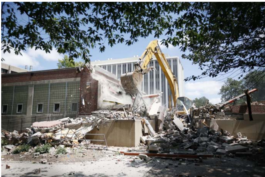
Demolition of Ferguson Hall
