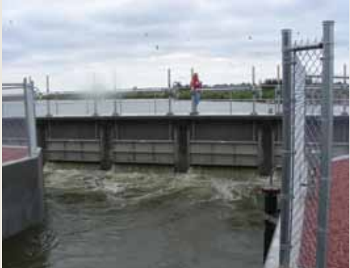
Pat Grant walks across the newly completed Taylor-Ord canal head gate near Taylor. The head gate had to be built to replace one that was washed-out by floodwaters in 2010.
